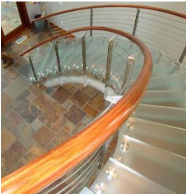
Circular Glass Stair in Place
