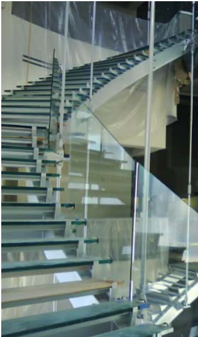
Glass Stair Case Under Construction
