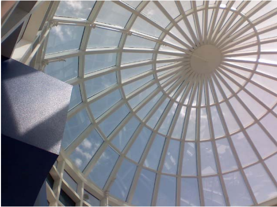
Interior photo of glass skylight
